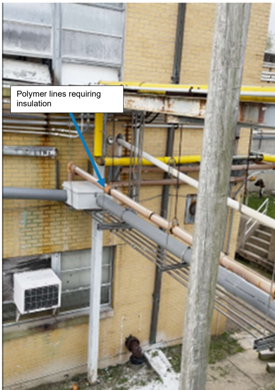
JHF-6. Polymer Feed Line: Proper insulation is missing and should be installed.
