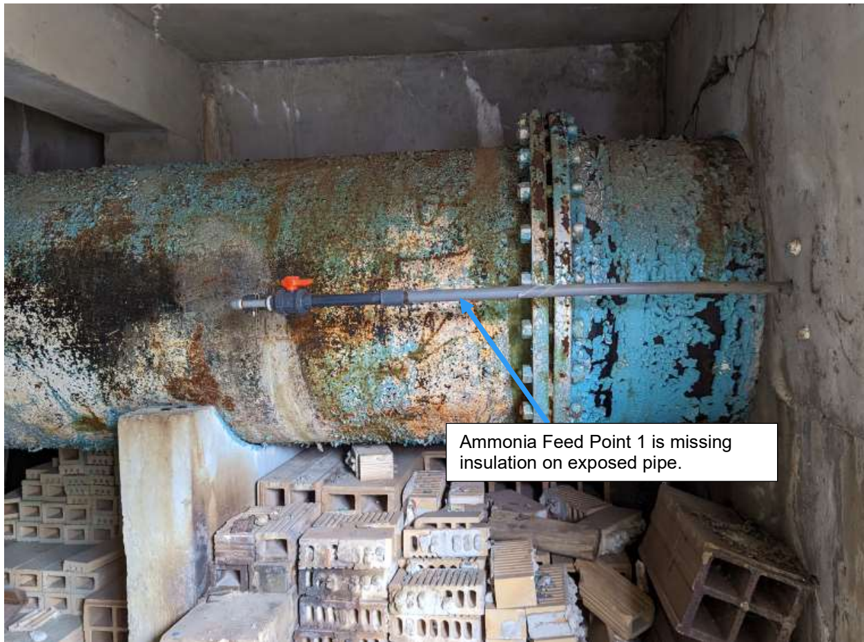
JHF-20. Ammonia Addition Point 1 on settled water line feeding Filter Building 2 needs insulation with heat trace.
