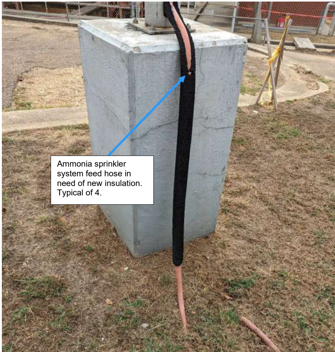
JHF-23. Water supply hosing to all the Ammonia sprinklers needs new insulation. There are currently 4 sprinklers with feed hoses in similar condition.
