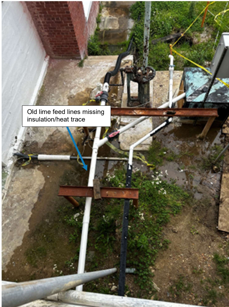
JHF-4. Old Lime Feed to High Service Pump Station: Proper insulation and heat trace is missing. Lines to be disconnected following implementation and acceptance of new Liquid Lime System in Fall 2023; no additional freeze protection recommended at this time.
