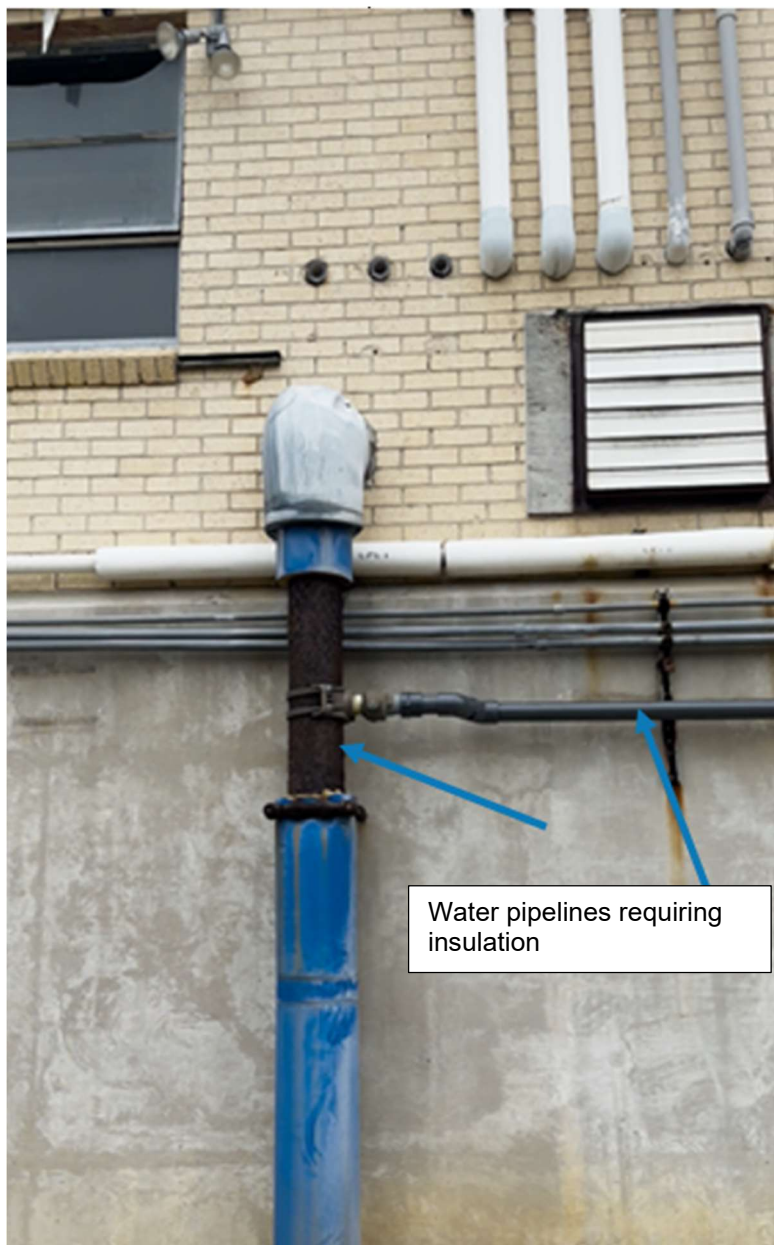
JHF-12. Recent Water Line Addition (Near Transfer Pumps): Proper insulation is missing and should be installed.
