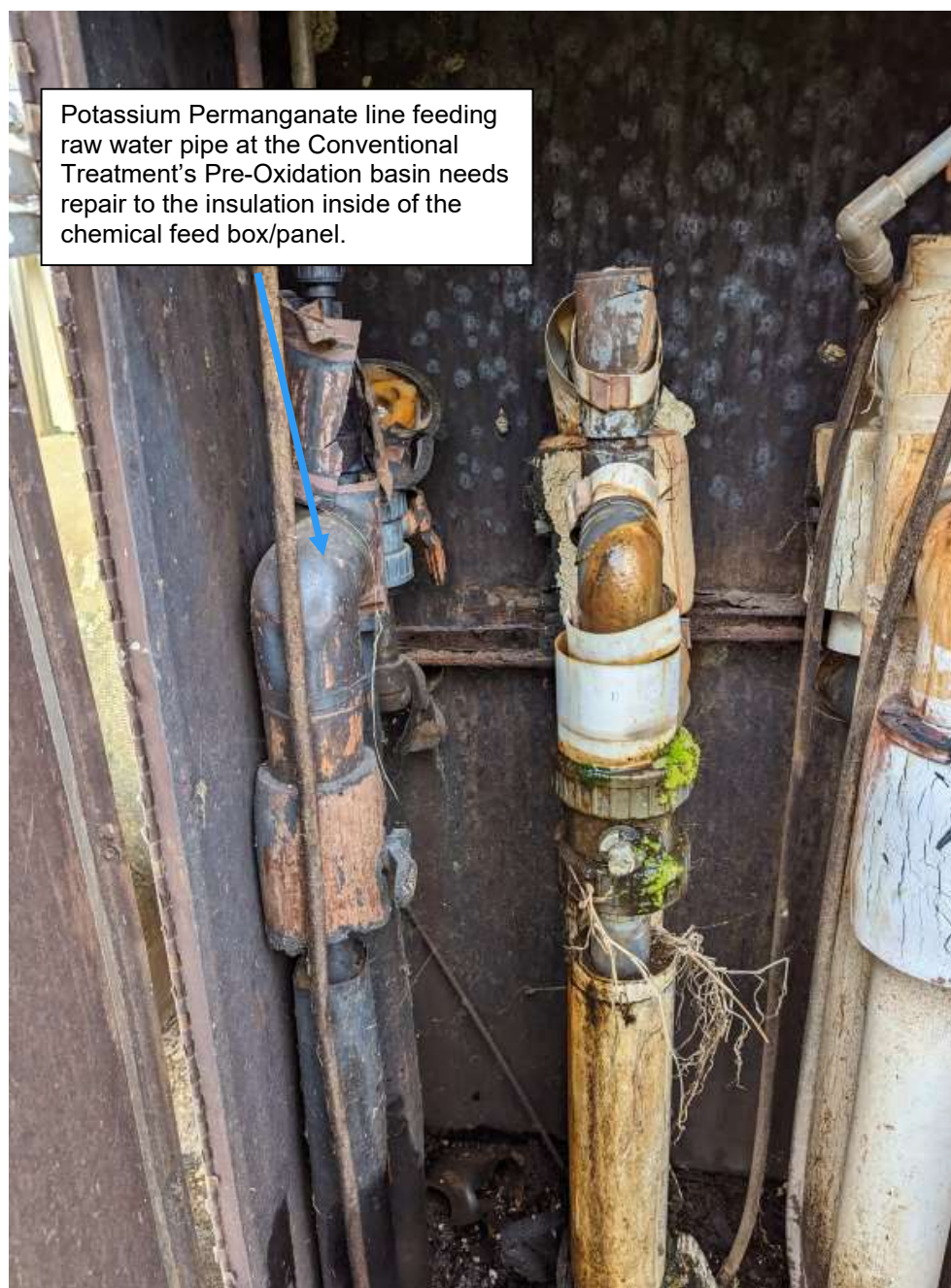
OBC-22. Potassium Permanganate line in chemical feed box at the raw water pipe headed to the Pre-Oxidation Basin for the Conventional Treatment train needs insulation repaired with heat trace. The other lines are abandoned.
