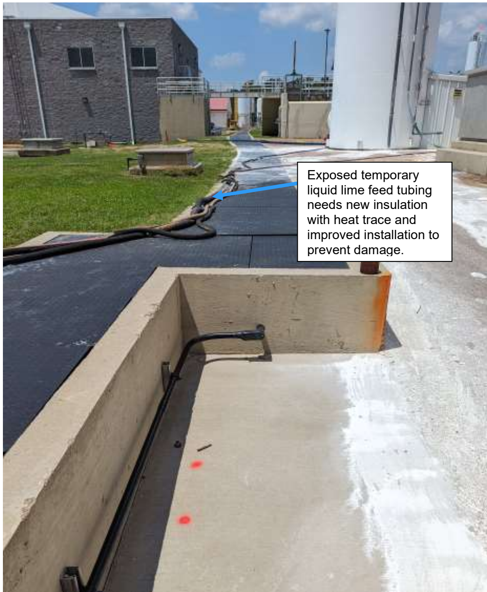
OBC-18. Temporary liquid lime feed lines to filtered water feed points need new insulation with heat trace and to be installed to provide additional protection to prevent damage.
