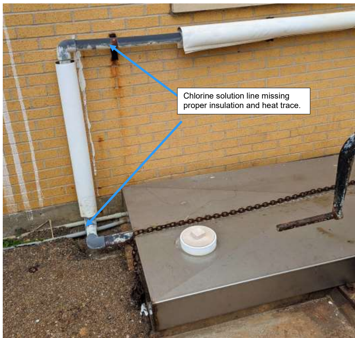
JHF-27. The chlorine solution line at post-sedimentation feed point needs insulation installed at missing locations and heat trace installed.
