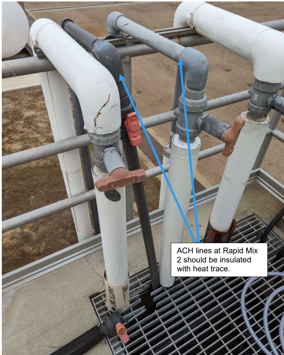
OBC-21. ACH lines need insulation/insulation repair and heat trace.
