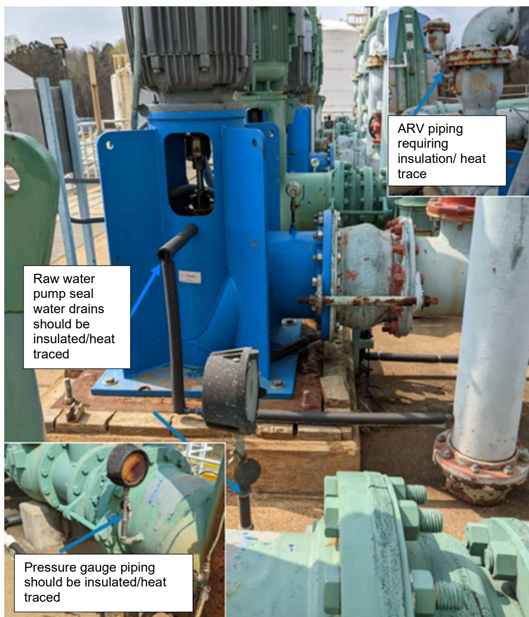
OBC-15, OBC-16, OBC-17. Raw Water Pumps: Seal water drains, pressure gauge piping, and air release valve piping need insulation and heat trace.
