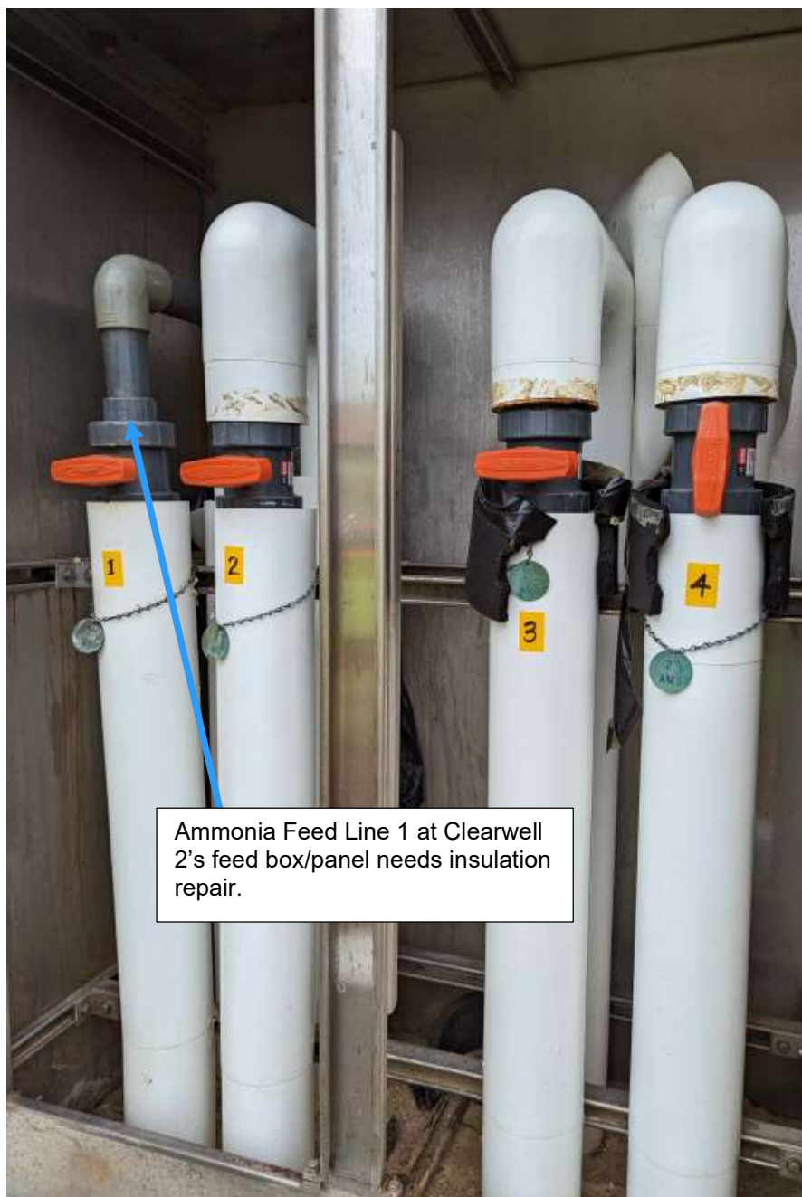
OBC-23. Ammonia Feed Line 1 at the Clearwell 2 needs insulation repair inside of feed box/panel.
