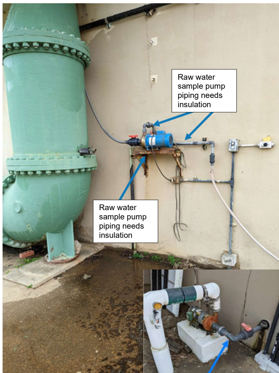
OBC-13, OBC-14. Raw Water Sample Pumps at Pre-ox Basin: Insulation and heat trace are missing.
