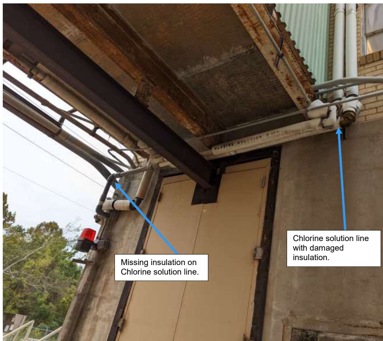
JHF-18. Chlorine solution line has damaged and missing insulation at several locations that needs to be repaired.
