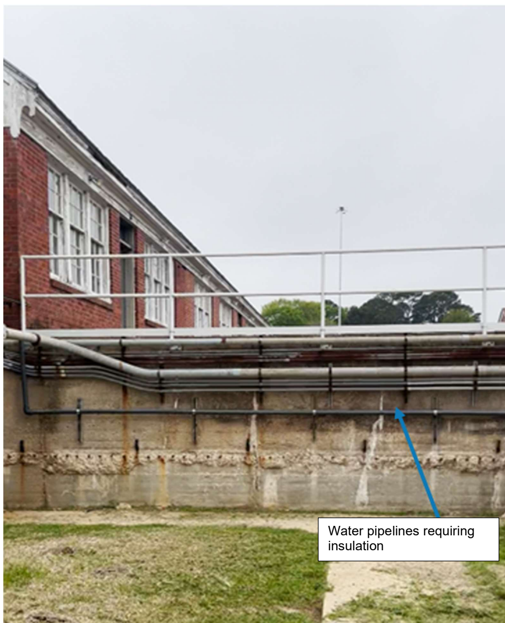
JHF-13. Recent Water Line Addition (Near Transfer Pumps): Proper insulation is missing and should be installed.
