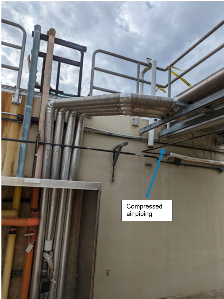
OBC-3. Compressed Air Pipe at Rapid Mix Heading to Soda Ash Silos: Used to clean out the silo dust filters; missing insulation could lead to condensation within pipe and introduce water to soda ash.
