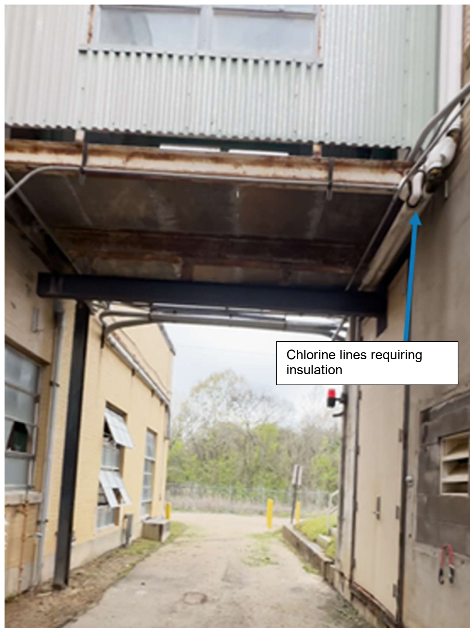
JHF-9. CP3 and CP4 – Prefilter Chlorine Feeds: Proper insulation is missing and should be installed.
