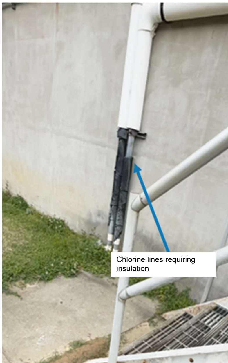
JHF-11. CP3 and CP4 – Prefilter Chlorine Feeds: Proper insulation is missing and should be installed.
