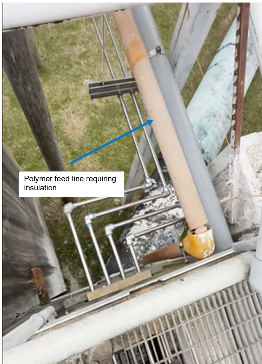
JHF-5. Polymer Feed Line: Proper insulation is missing and should be installed.
