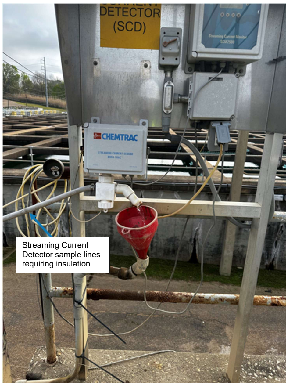
JHF-1. Streaming Current Monitor at the Flume and Turbidimeter for Sediment Basins: Sample lines need proper insulation installed.
