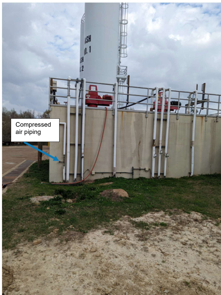
OBC-2. Compressed Air Piping on Rapid Mix Wall: Missing insulation could lead to condensation inside line.
