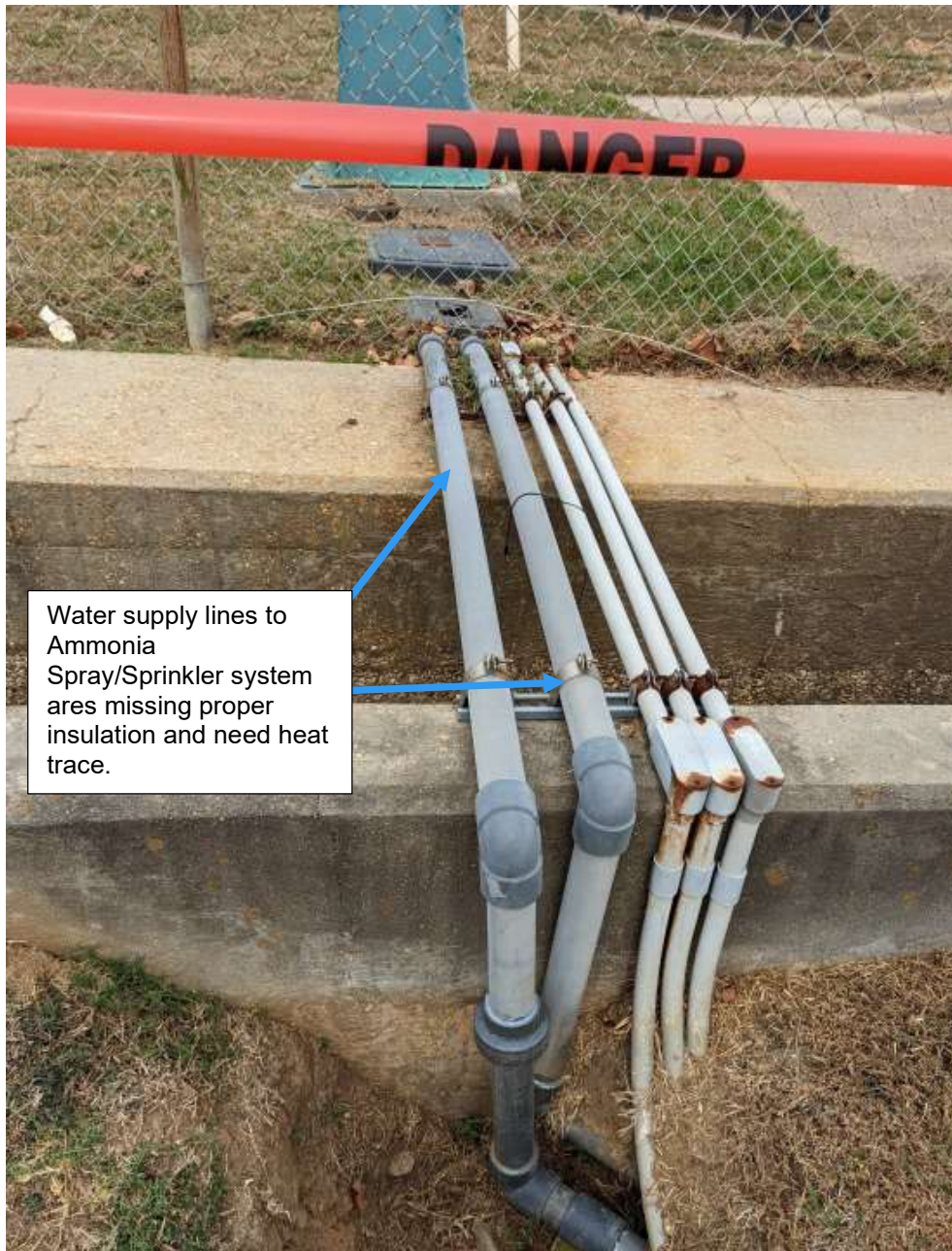
JHF-22. Water supply lines to the Ammonia Spray system/sprinklers need proper insulation with heat trace.
