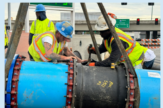
Crews complete valve and pipe replacements at Northside Drive and I-55.
