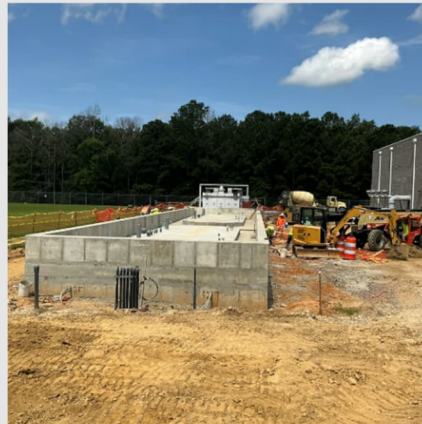
100'x25' Concrete Foundation Completed for Liquid Lime Silo's
