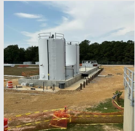
20,000-gallon Liquid Lime Silo's and Metal Building Installed
