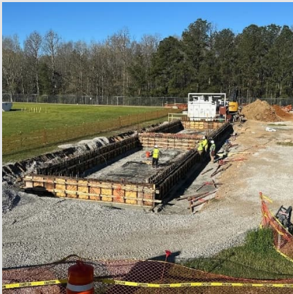
Grading, rebar, formwork prepared for Concrete Foundations
