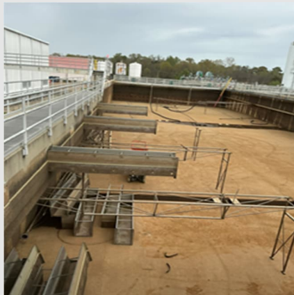
Demolition of Sediment Basin 3 in preparation of new launders and settlers.
