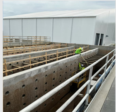
Baffle walls raised for increased capacity.
