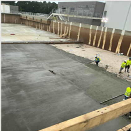
Pouring new concrete pad floor in basin in preparation of new sludge collection system.
