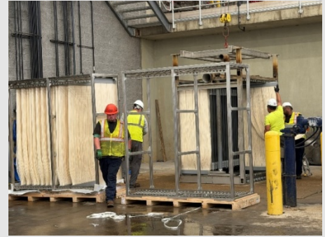
Operations staff install new membrane trains at O.B. Curtis Water Plant
