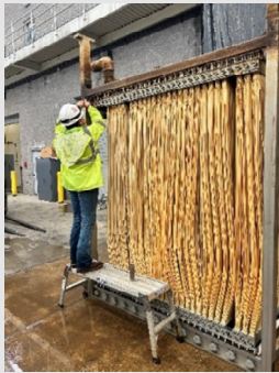
Operations staff remove old fibers from membrane cassette
