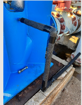
Insulation installed around exposed pipes
