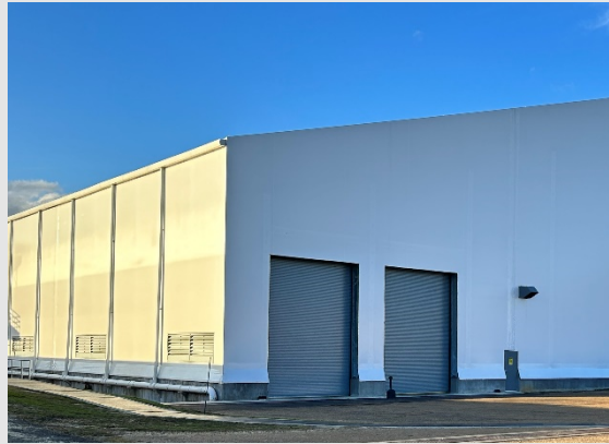
Winterization through the full enclosure of the membrane building
