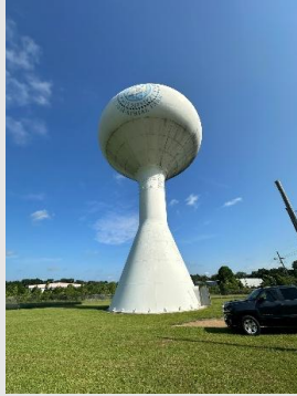
Industrial Park water storage tank
