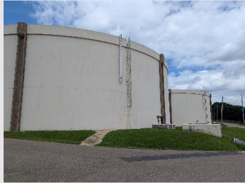
Finished water ground storage at J.H. Fewell Water Treatment Plant
