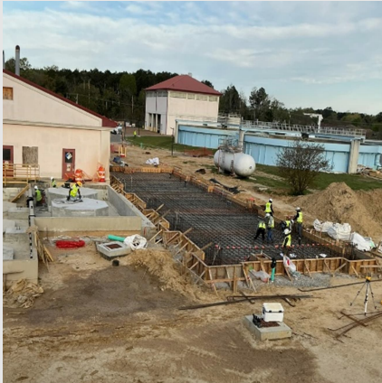
Sodium Hypochlorite Containment being prepped for concrete
