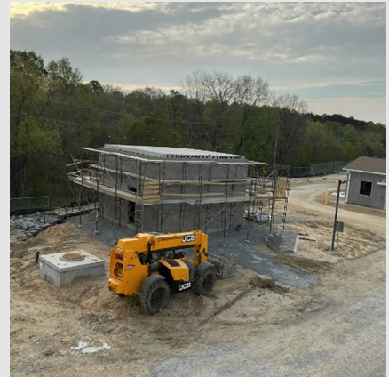
Raw Water Electric Building foundation, walls, and roof panels.
