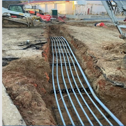
Underground electric conduit being installed.
