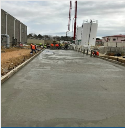
Concrete Apron in front of the Liquid Lime Silo's
