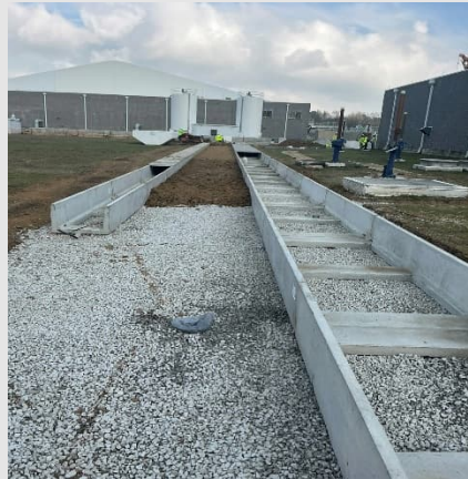
Chemical Trenches being installed for piping
