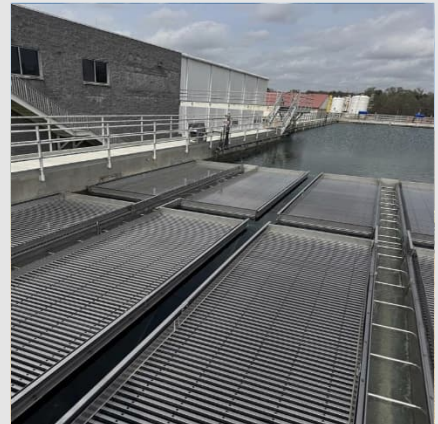
New plate settlers installed and operational in Sediment Basin 3
