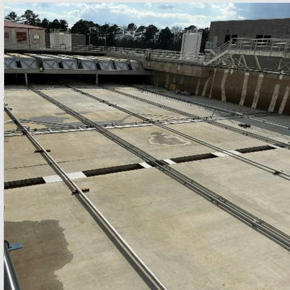
Installing sludge collection equipment in Sediment Basin 3
