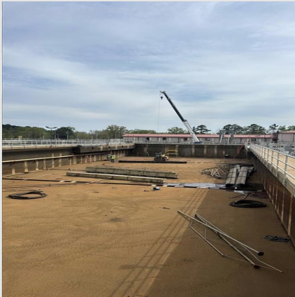
Demolition of Sediment Basin 2 launders, supports, and sludge collection system
